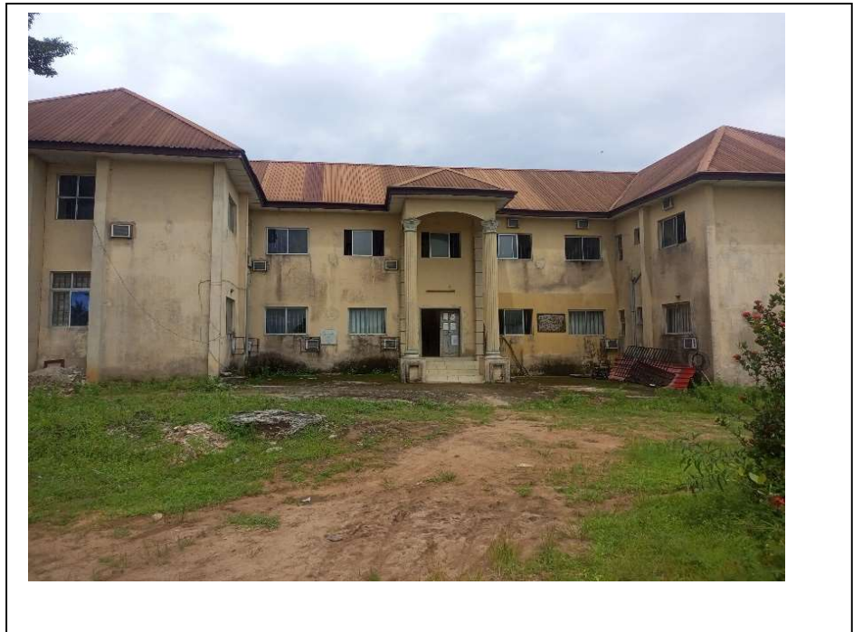
Temporary SESET Office (Okiro Building)
